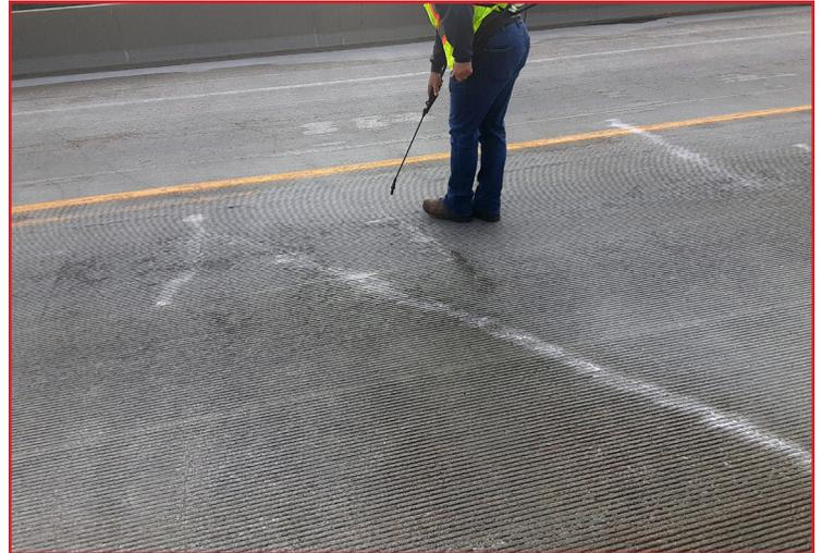
4. Begin by flooding all cracks. This includes cracks less than 5/64" (2.0 mm) and also cracks that have been routed or ground. The purpose of this spraying is to ensure that all cracks have a sufficient amount of waterproofing material within them. In this situation more is always better.
